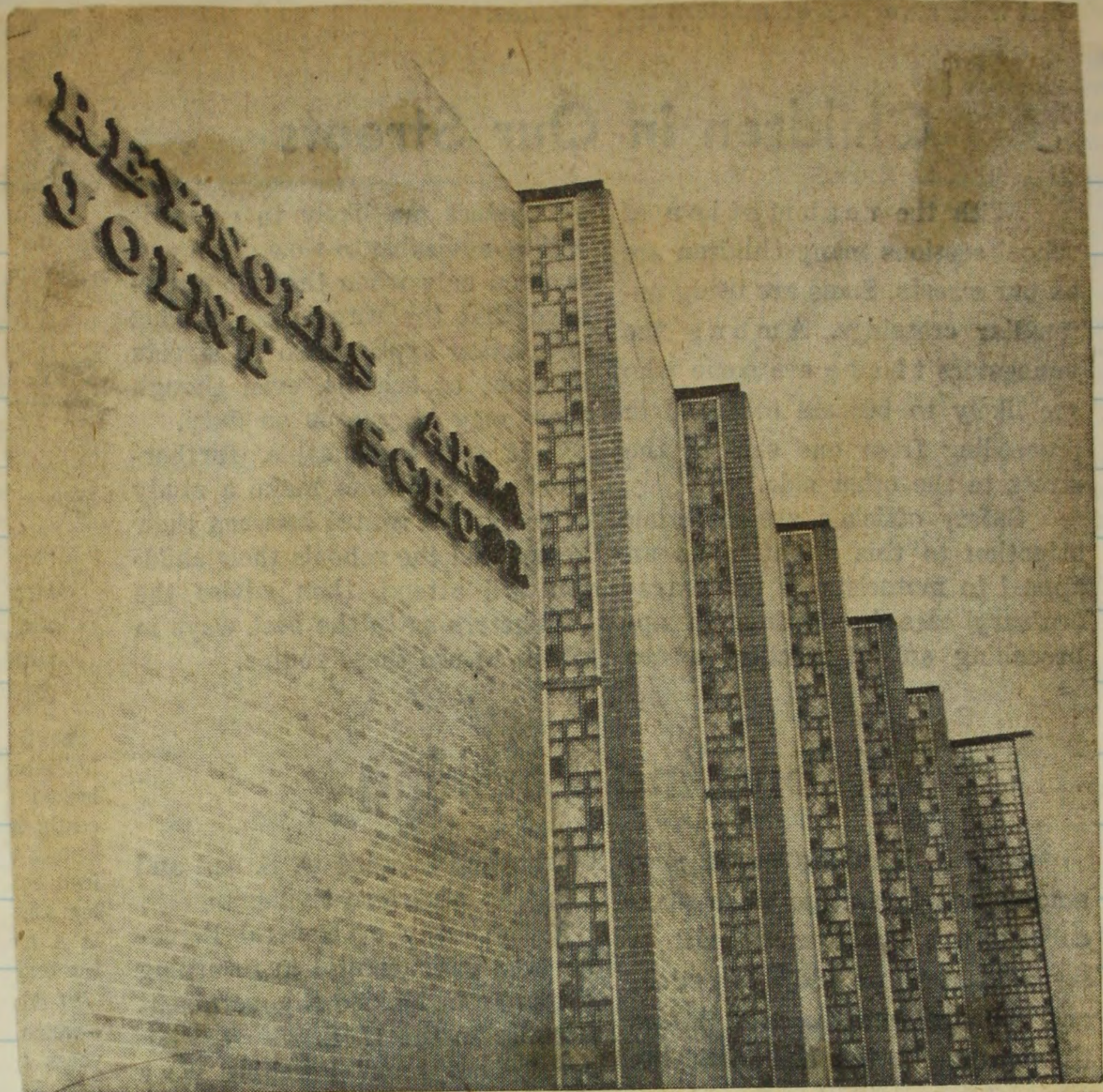
EXTERIOR AUDITORIUM WALL —Offsets with portions comprised of clear and colored glass bricks provide a unique appearance for the exterior wall of the school's auditorium.
